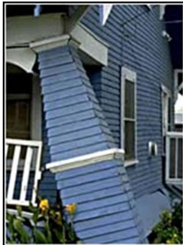
Figure 27 Structural Earthquake Damage
